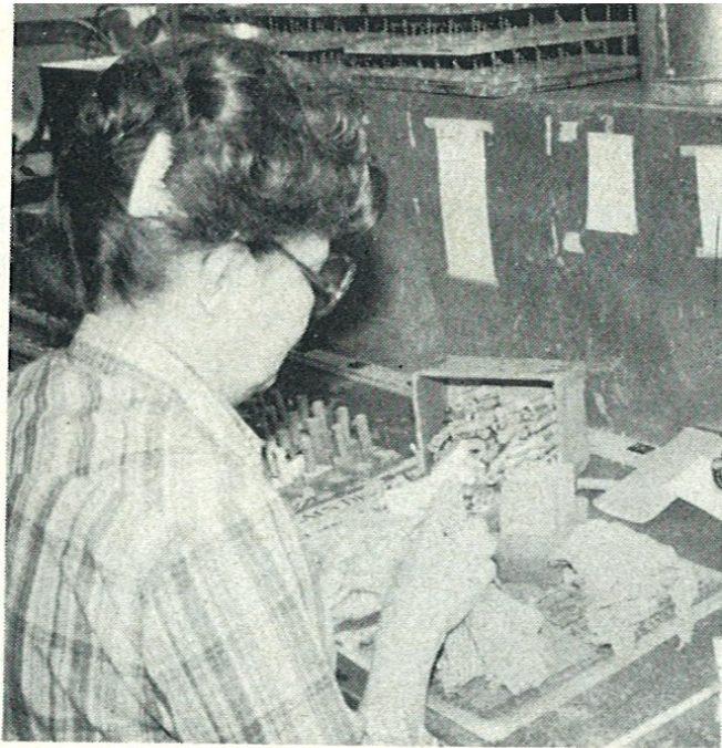
Above left: Parma resistors being finished off with 'refractory wash'. Above right: the storage area for the resin bodyshell formers. Below: Parma resistors actually being machine wound. Far right: Just part of the shipping and storage area from where Parma products are distributed all over the world.
